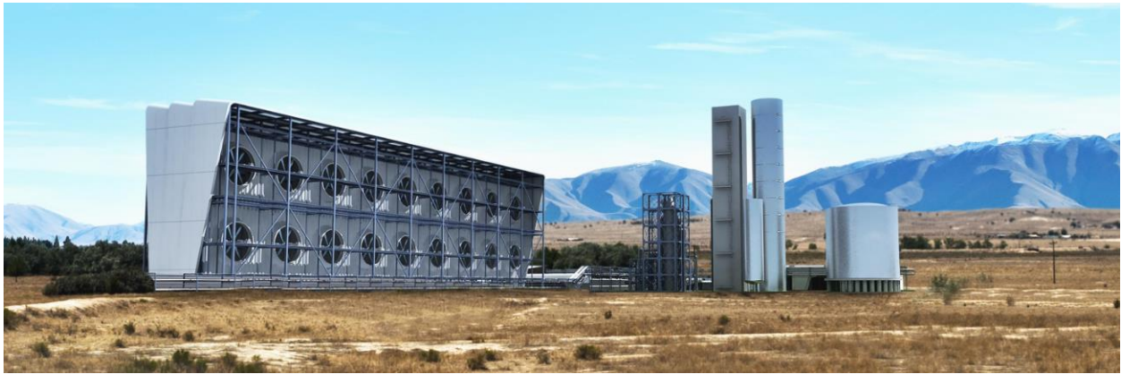
Carbon Engineering Direct Air Capture
